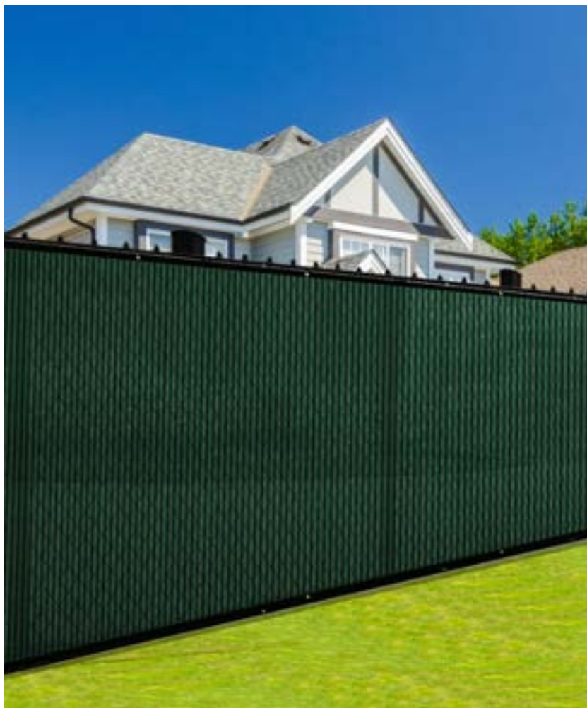
Figure 2-6: Example of silt screen fence.
