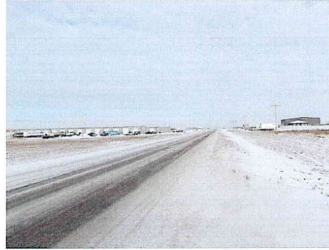
Looking North on Gravel Pit Rd.
